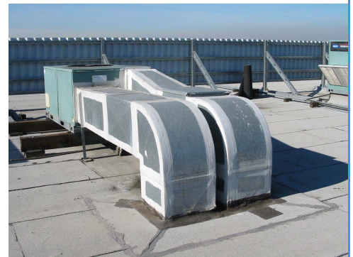
Side discharge with exposed ductwork
