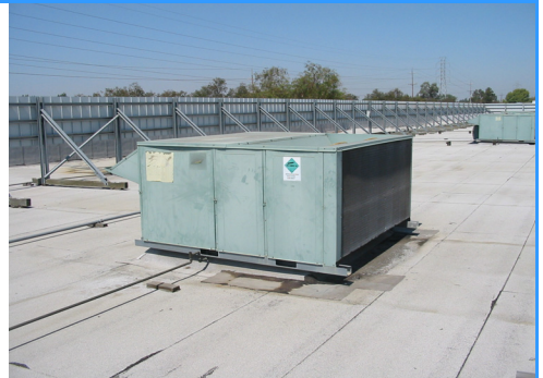
Bottom discharge-no exposed ductwork
