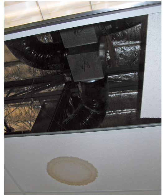
Interior view of leak under return air plenum
